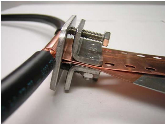
**Figure 11: Completed Strap Assembly.**
